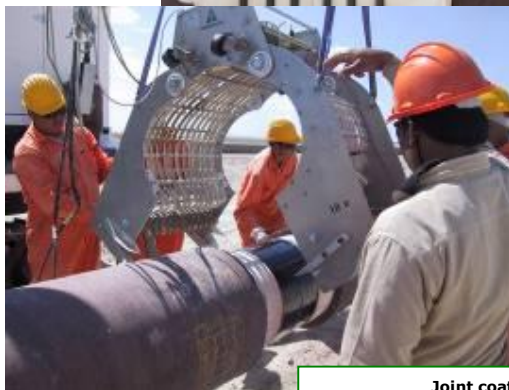
Joint coating preheating
