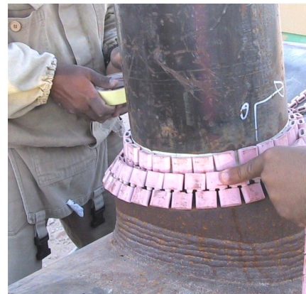
Heat treatment for stretch welding through electric resistances
