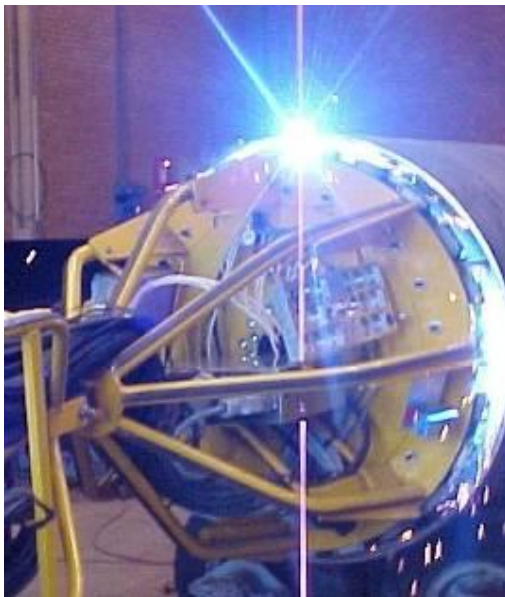
Pipe coupler with automatic internal welding
